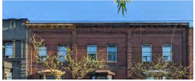
Figure 57: 1468A-1472 Queen Street West are representative examples of properties with a flat roof.
