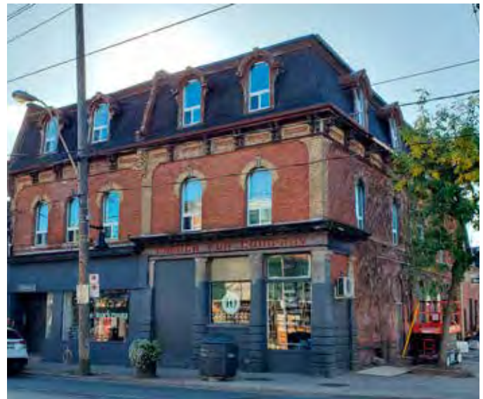
Figure 38: 1267 Queen Street West is a representative example of the Second Empire style.
