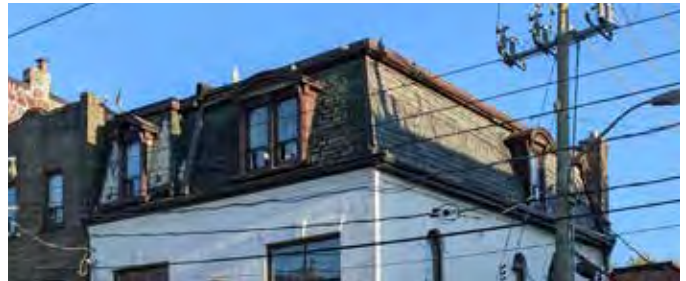
Figure 58: 1402 Queen Street West is a representative example of a property with a mansard roof.
