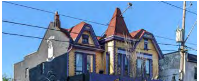
Figure 59: 1255 Queen Street West is a representative example of a property with a roof that has multiple gables.
