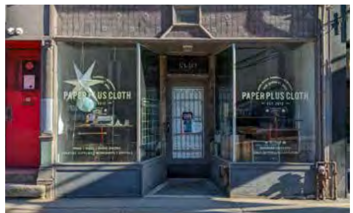
Figure 64: 1340 Queen Street West is a contributing property with a historic storefront.
