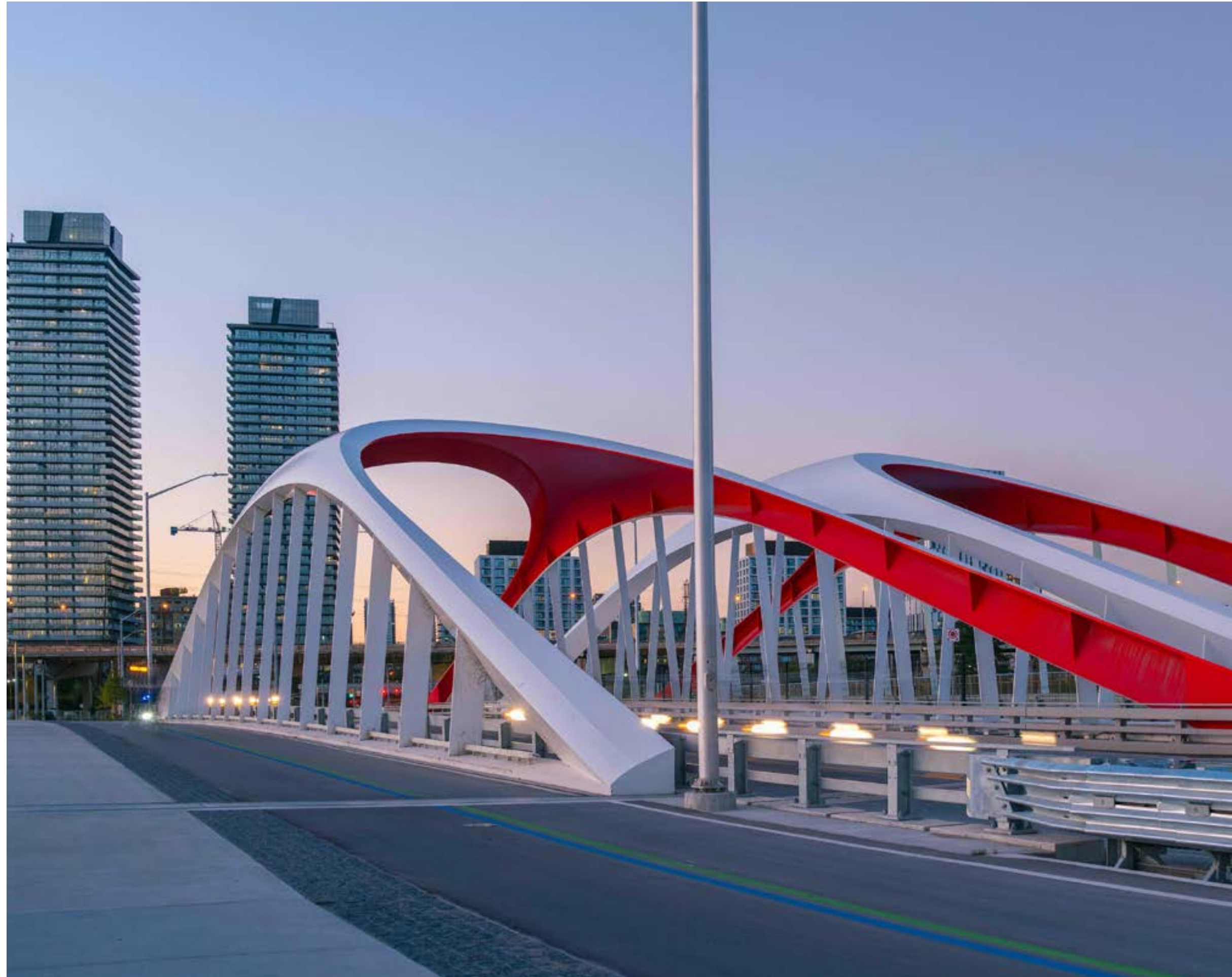
Port Lands Bridges, Photo credit: Jonathan Bacolor
