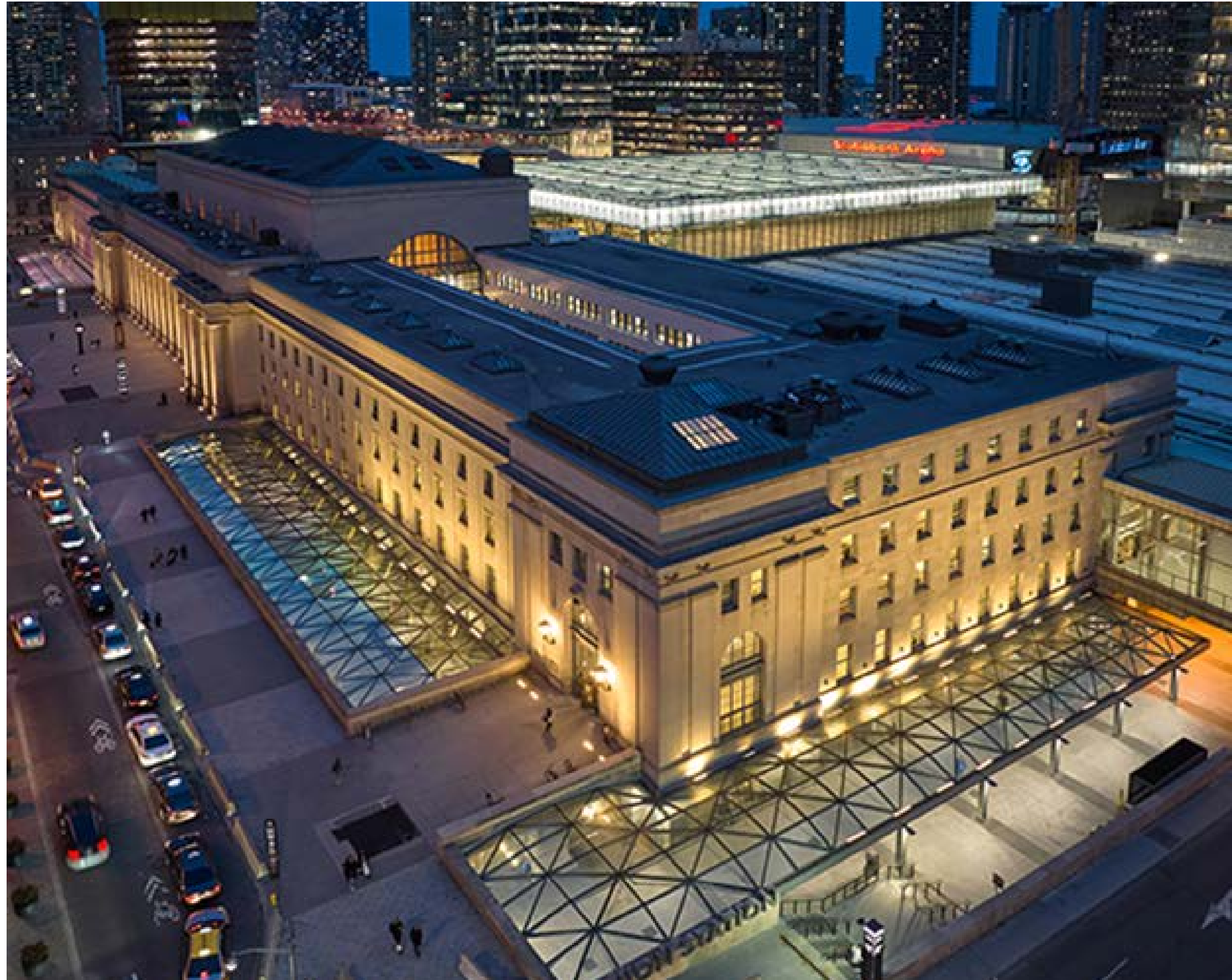
Union Station Revitalization, Photo credit: Doublespace Photography
