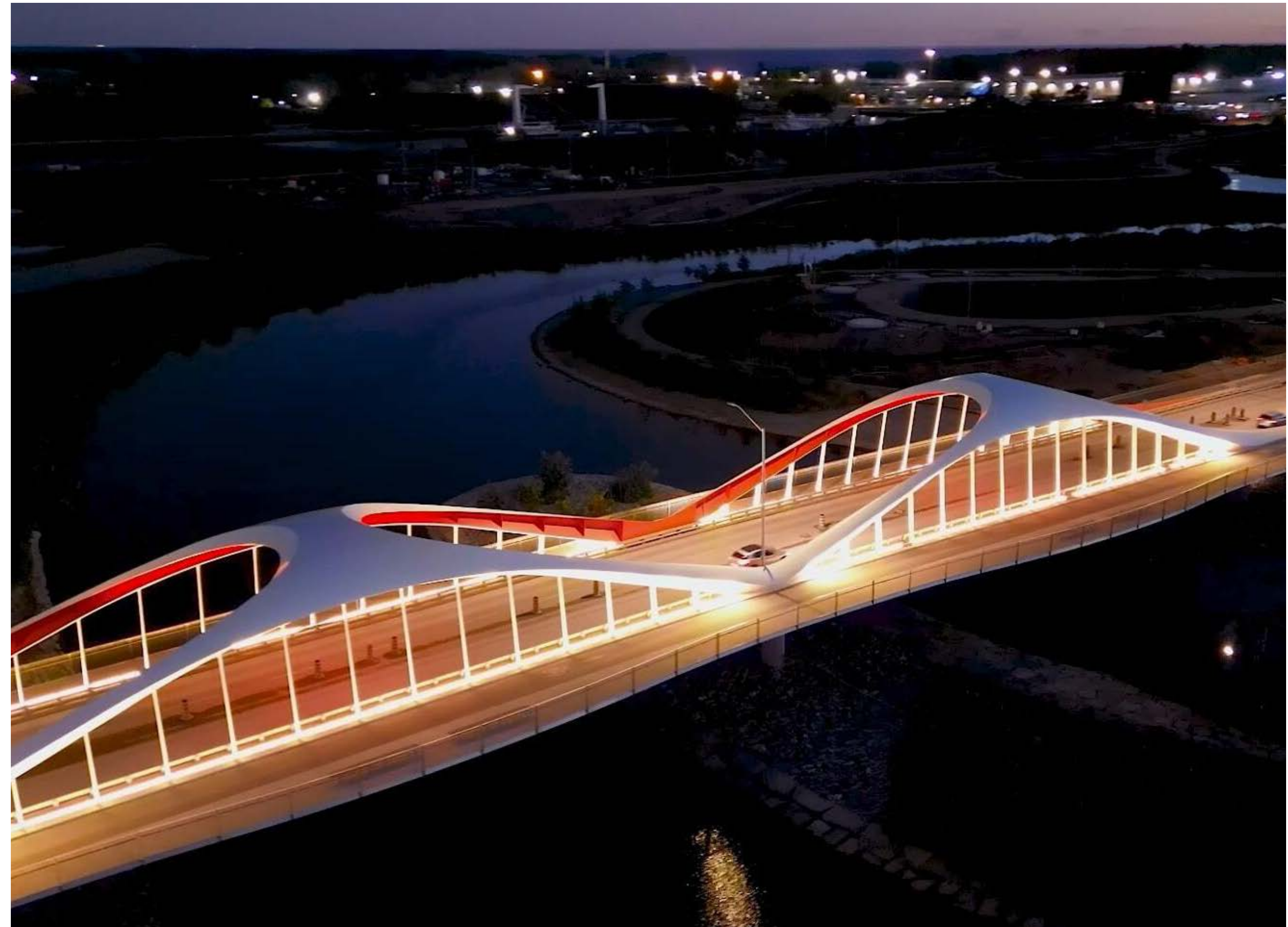
Port Lands Bridges, Photo credit: Olu Joseph
